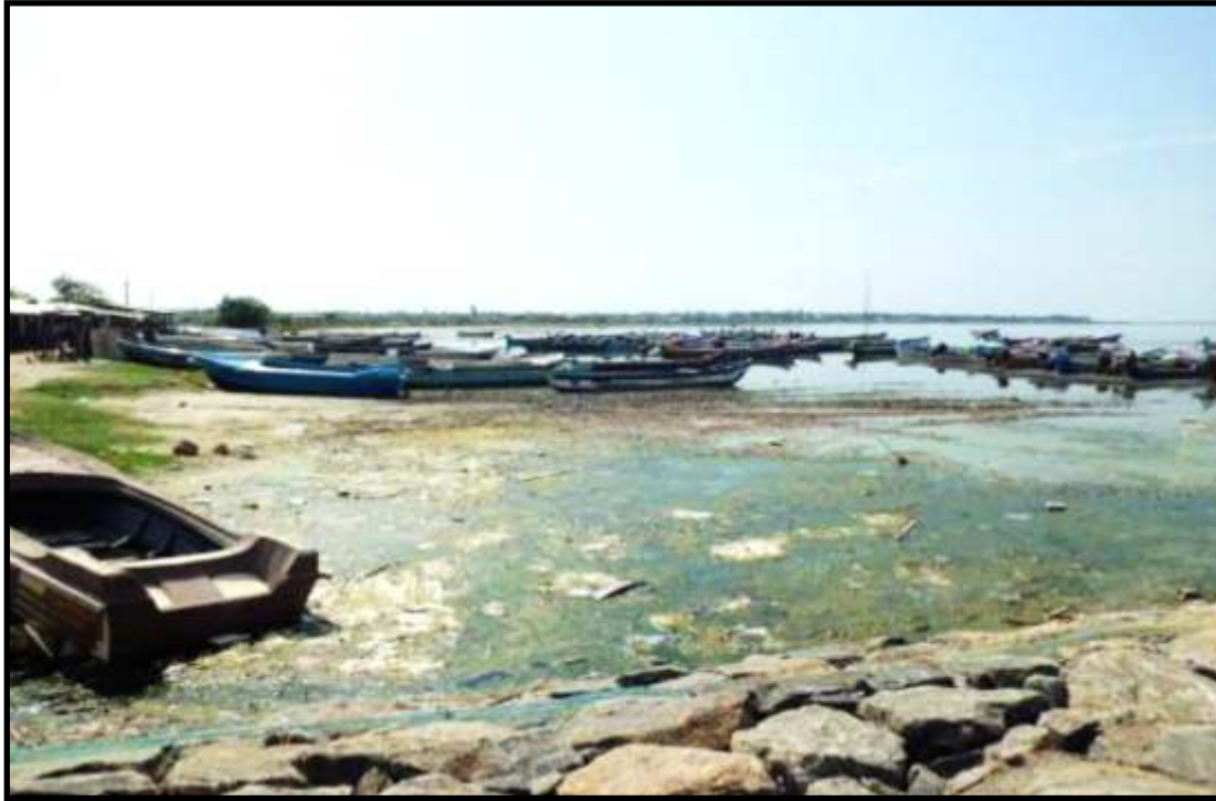
Plate I : Landing centre at Kakkaithivu
