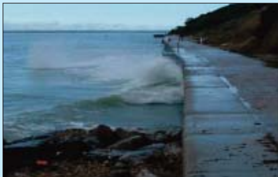
A Seawall replaced the shoreline
